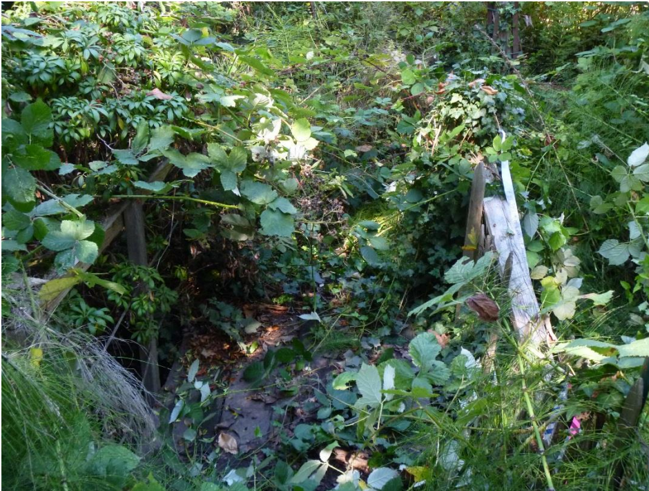
Figure 4. Wooden bridge over manmade berm, between Wetlands B and C
