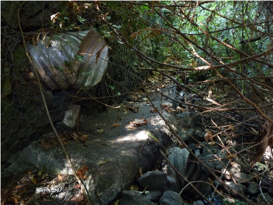
Figure 2. Watercourse A exiting Wetland C, with culverts under Island Crest Way
